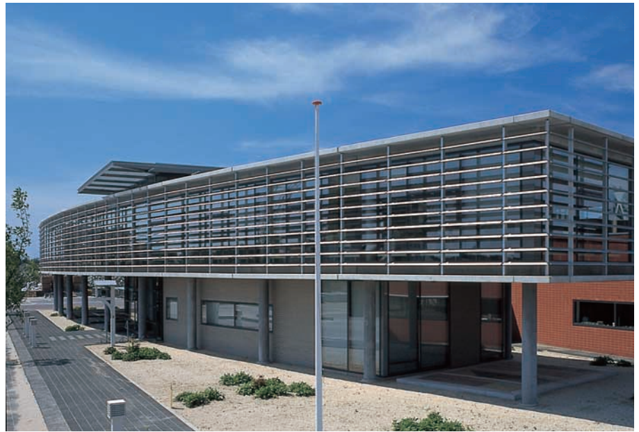
Material centre & Omegam, the Netherlands
